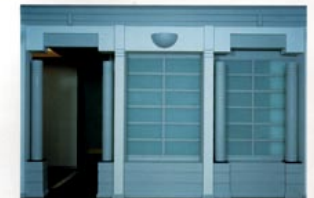
Deborah Natsios' interior features painted columns without capitals or any structural function. (right) suspended glass doors allow to screen the living room from the foyer (below)
